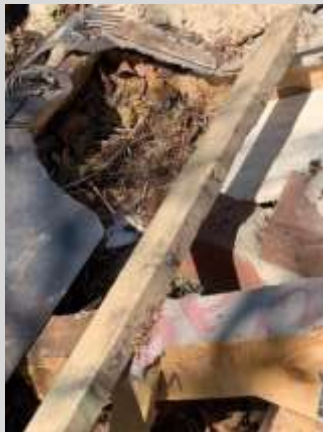
Cleared the squirrels' nest and re-roofed the garage
